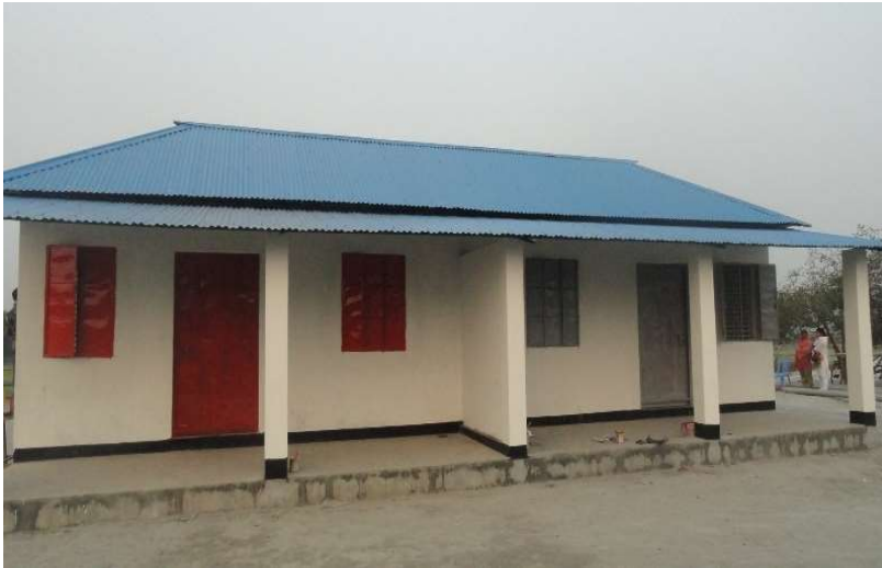
Figure 5: Resettlement House (2 units) Source: Author (2014)
