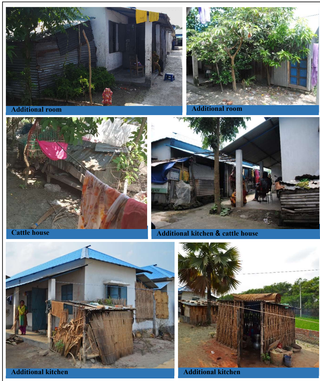
Figure 9: Current scenario of additional structure Source: Survey 2018
