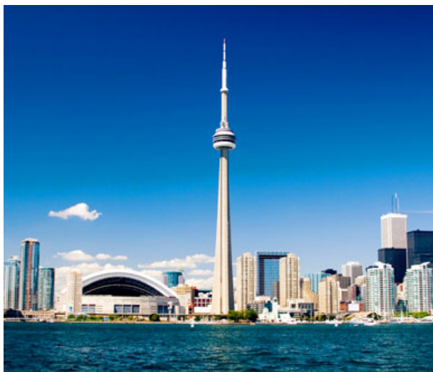
CN Tower, John Andrews Architects, Toronto, 1976.
