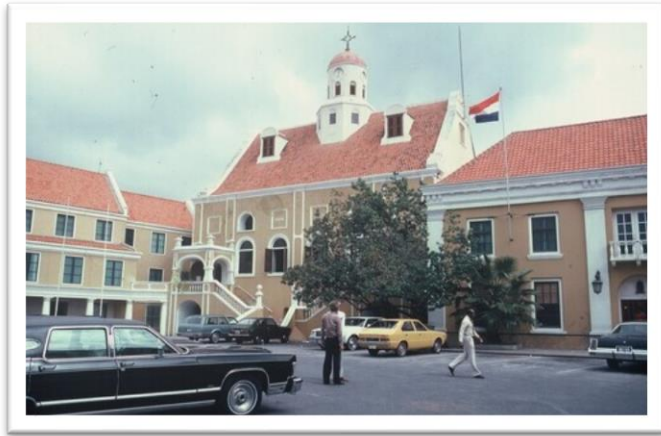
7.12: De Jonge, 'Courtyard of Fort Amsterdam with the fort Church' (1980-1983).
