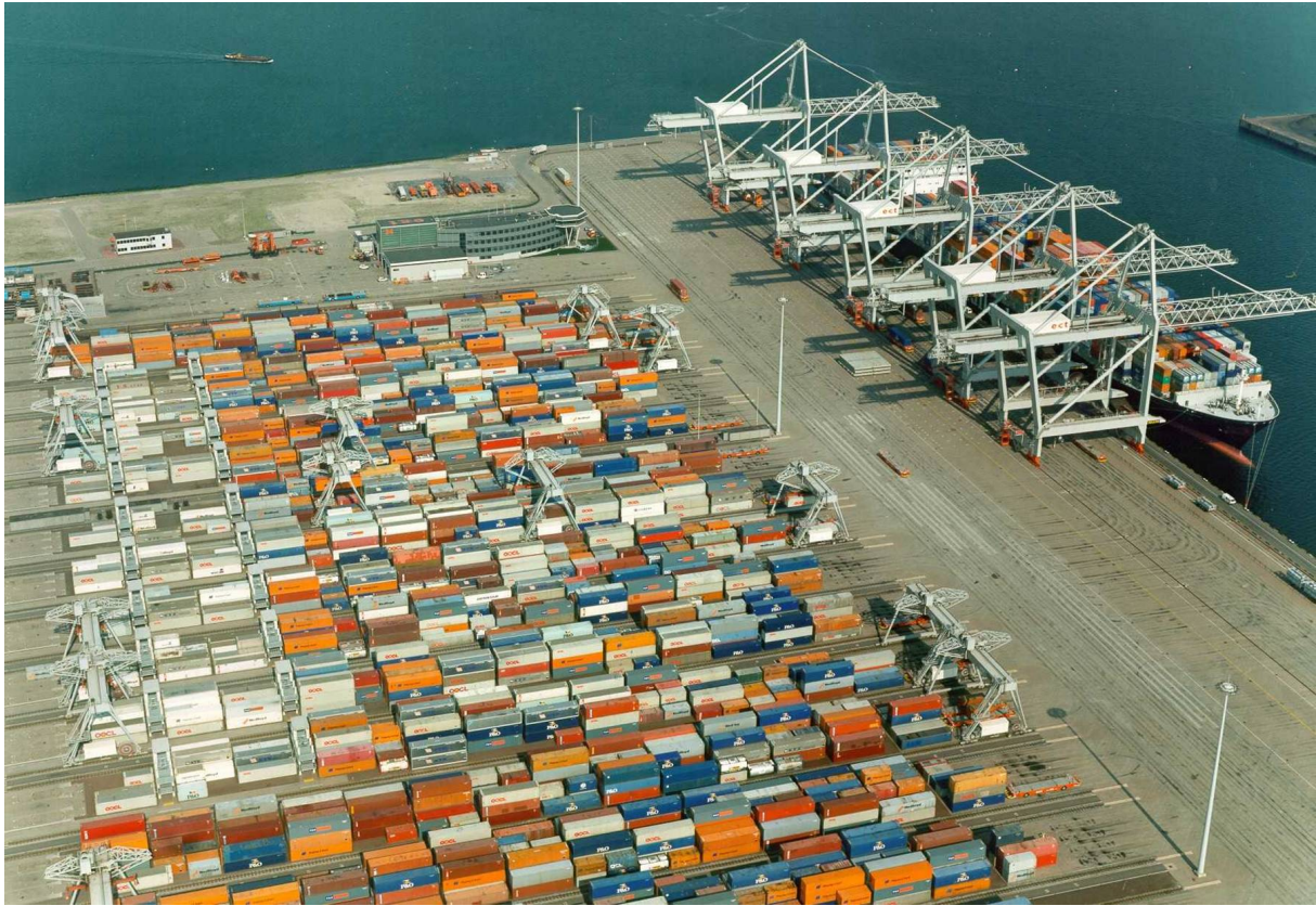
Figure 3.2: Aerial overview of the ECT terminal in the port of Rotterdam. Source: [5]
