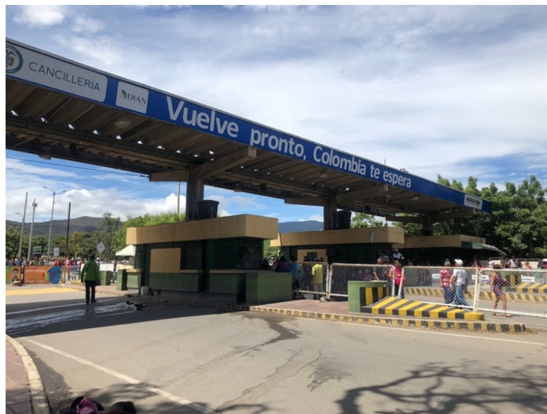
Figure 1 'The International Simon Bolivar Bridge'
