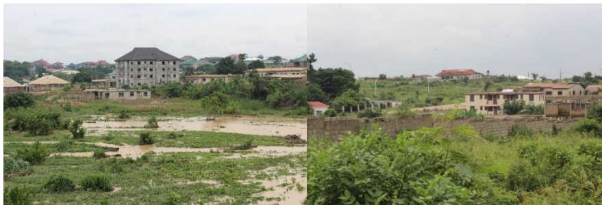
Photo 3. Images of ongoing settlement construction within green spaces in Asokore Mampong.
