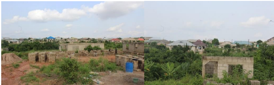
Photo 4. Images of ongoing settlement construction within green spaces in Kwabre East.
