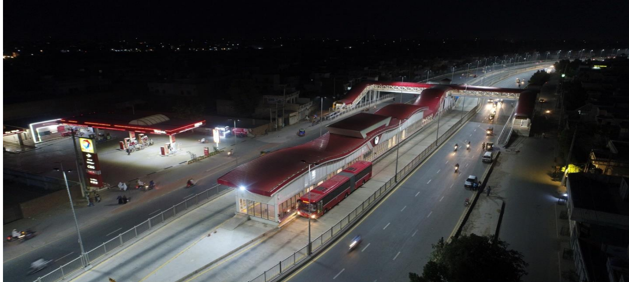
Figure 1. Aerial view of a Metro Station (photo courtesy: www.paksteel.com )
