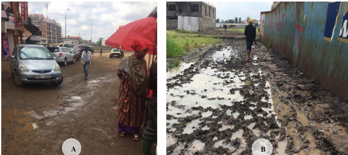
Photograph 1: Road conditions in Ruiru Bypass Zone
