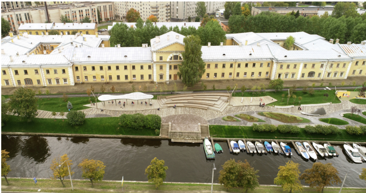
Photograph 1: The central part of the development of the Karpovka river embankment. 'Before' and 'after.' (Retrieved from Landscape architecture and design agency "Neskuchny Sad", 2019).
