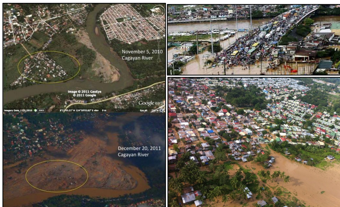
Photo 2. Damages of TS Sendong in Cagayan de Oro City
