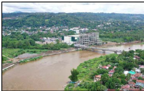
Photo 1. Unfinished mall beside the Cagayan river (abandoned because it submerged during TS Sendong)
