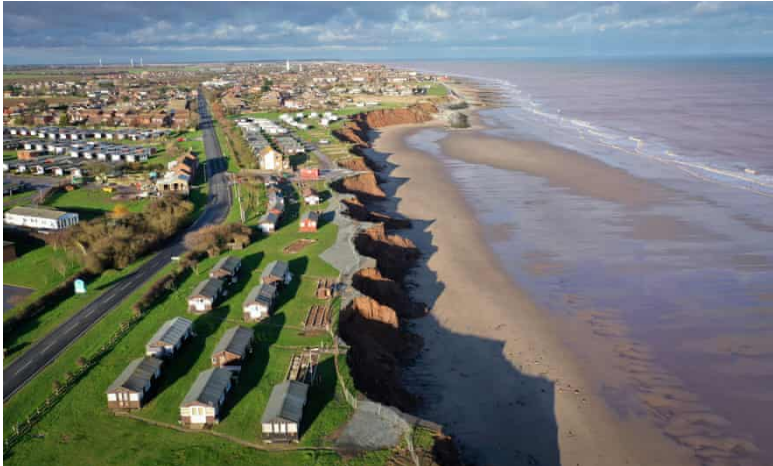
Figure 7; Holiday housing abandoned due to coastal erosion in Yorkshire, UK (Halliday, 2020)
