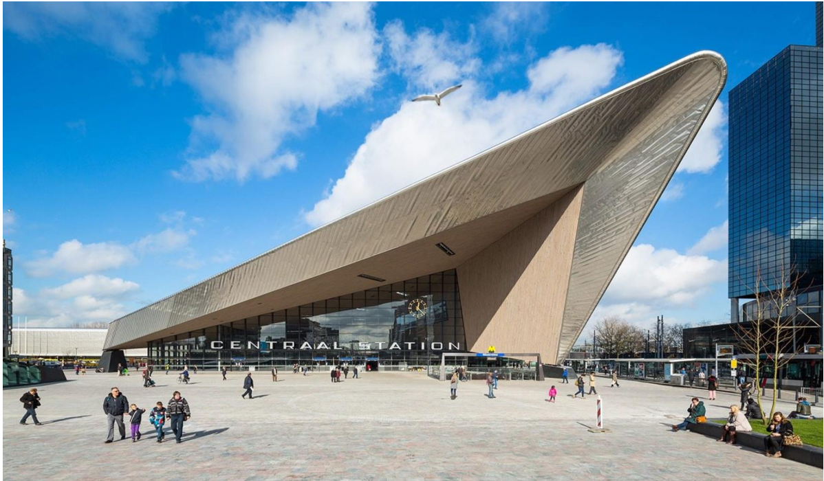
Figure 4.12 Rotterdam Central Station (Team V Architectuur, 2014)
