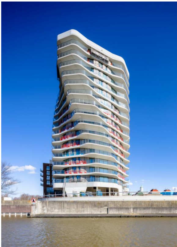
Figure 4.19 Manhattan tower in Roermond (Gijssels, 2020)
