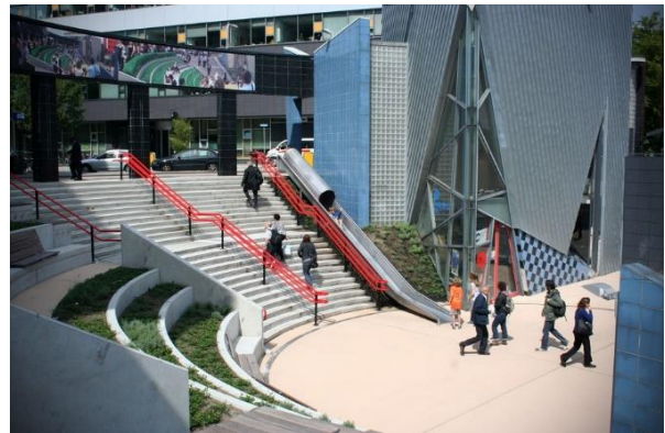
Figure 2.5 Slide in train station Utrecht Overvecht (DUIC, 2016)
