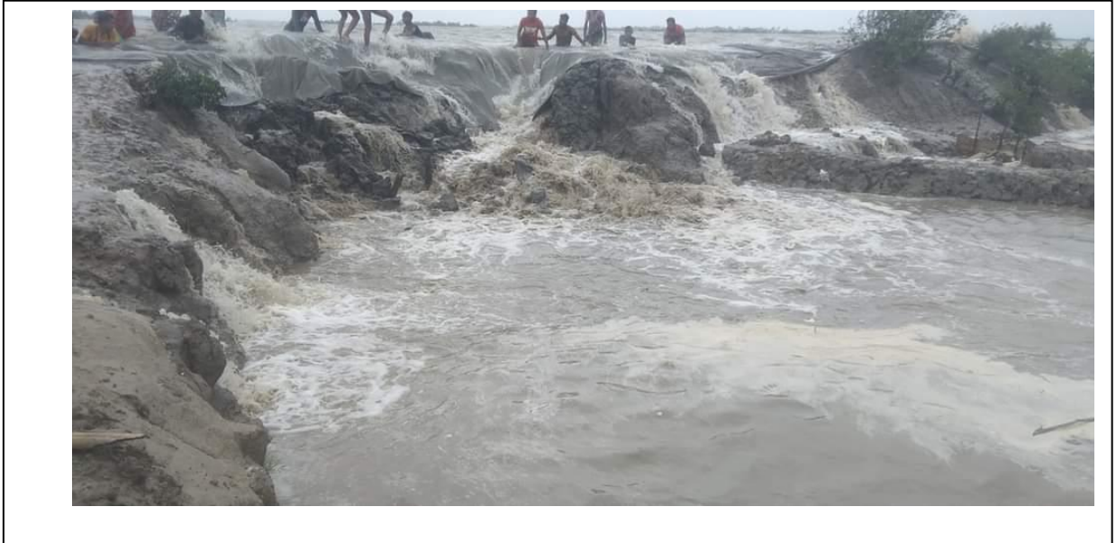
[Figure 2: Collapse of embankment during cyclone Yaas ]
