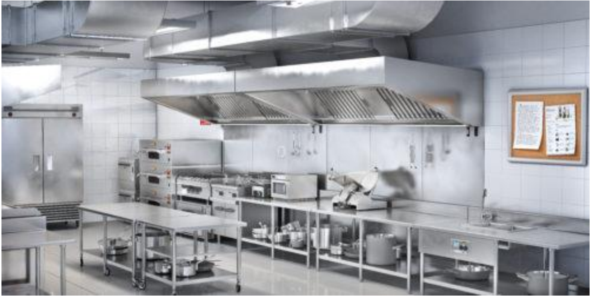
Figure 3.1: Kitchen 1 (clean kitchen)
