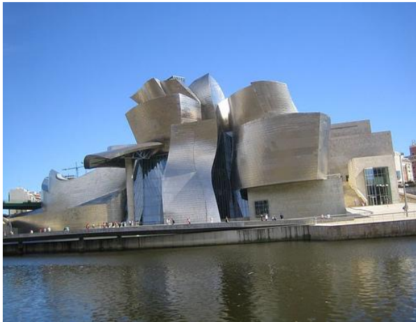
Figure 1.1 Guggenheim Museum Bilbao
