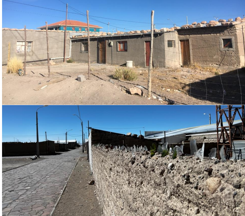
Figure 20. Fences and Walls
