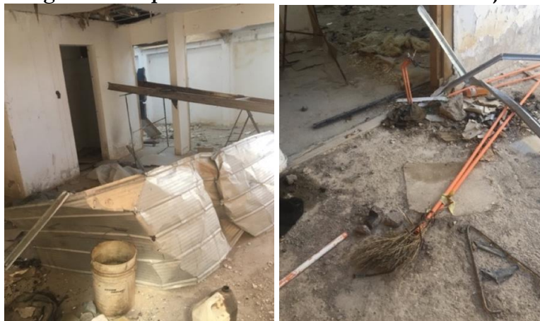
Figure 19. Improvised Shelters at Abandoned Project
