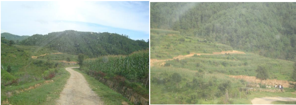
Road constructed using bulldozer in the watershed area (Picture: Author)
