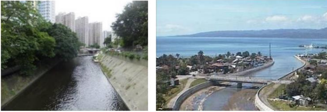
Figure 10 An example of drainage channels in urban areas, Source: FFC, MOWR, Annual Flood Report 2020
