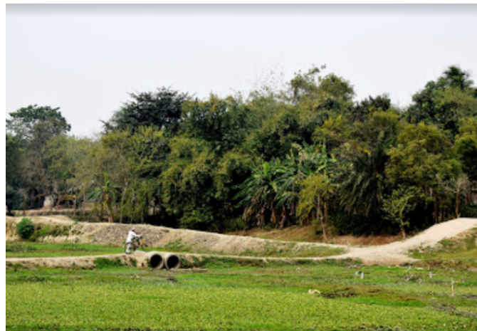
Photograph 9: Anjana river in rural areas showing illegal road over river with river flowing through pipes (Source: Author)
