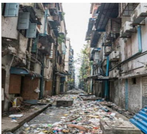
Figure 2: Alley Condition before 2016
