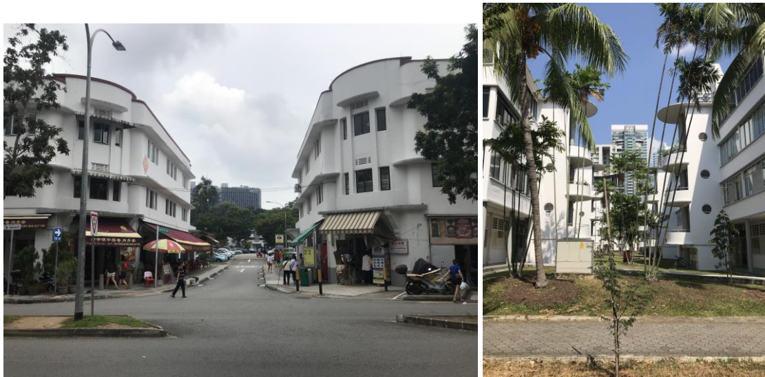
Figure 6 Conserved pre- and post-war SIT blocks at Tiong Bahru (Source: Author's own)
