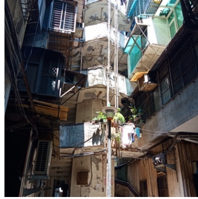
Figure 4. Nan Chi Chang public housing buildings.
