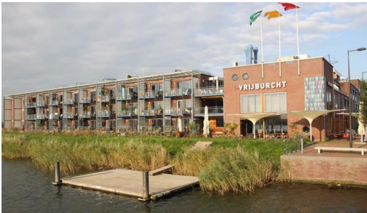
Photograph 1: Vrijburcht design by (CASA Architecten).
