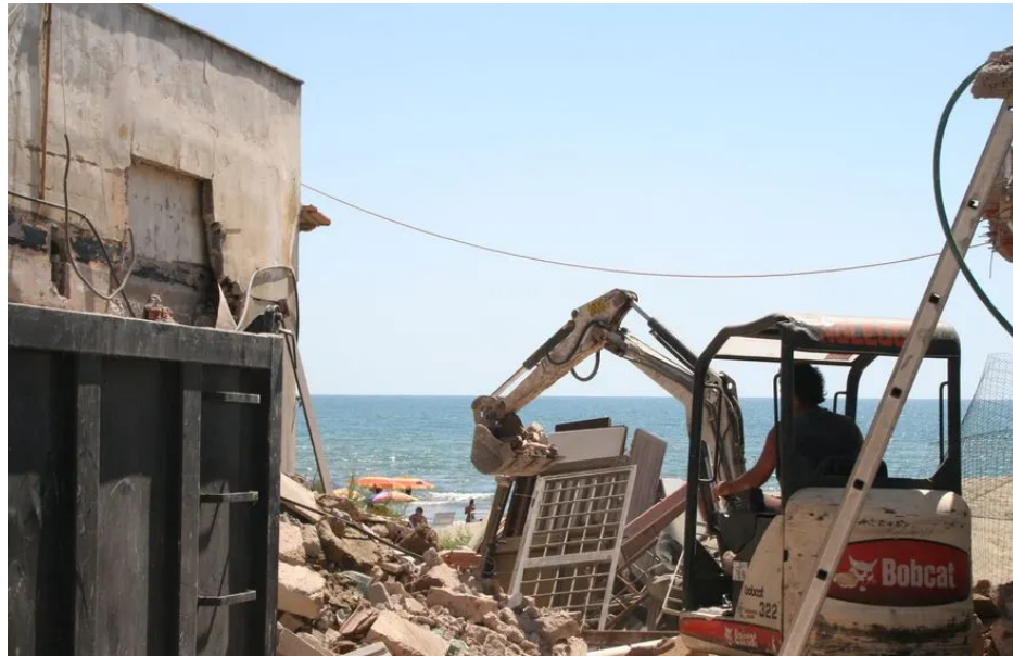
Figure 10: Bulldozing an unauthorised construction in Torre di Gaffe, Licata, Sicily
