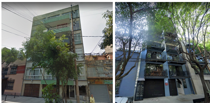
Picture 1 Case 1 projects. Ozuluama 20 before (2017) and after (2023).
