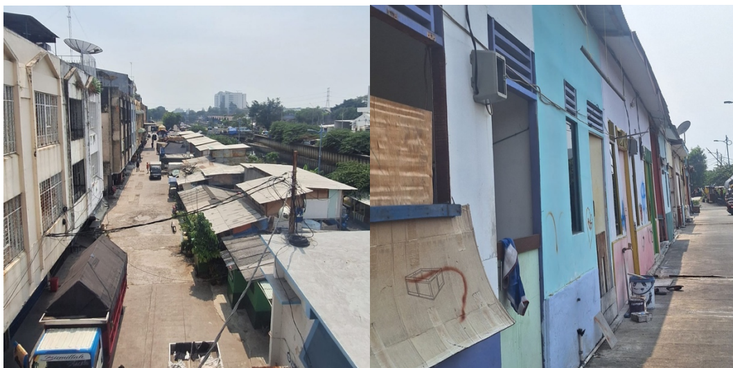
Left: Shophouses and de facto area of Kunir; Right: Temporal housing ( huntara )
