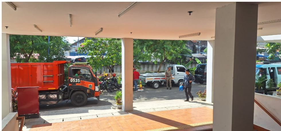
Kampung Kunir built in the same area of the old kampung . Front view: Tributary of Ciliwung River (behind riverbank wall), new Inspection Road which become the reason of eviction in 2015
