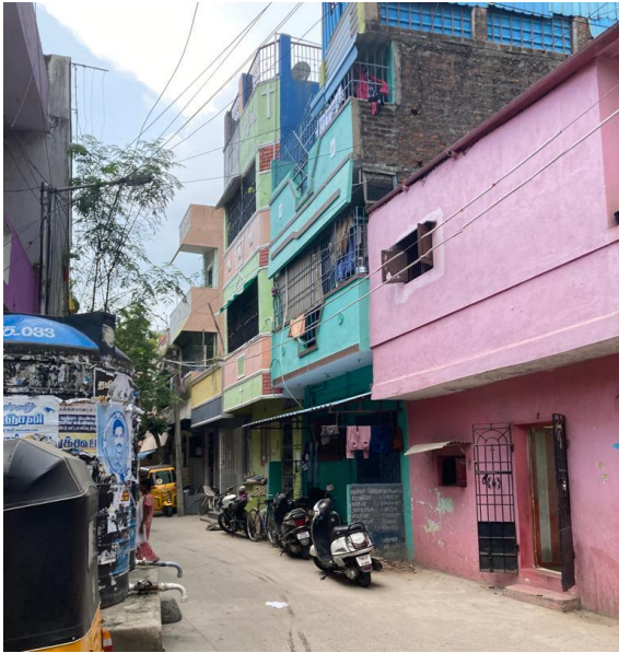
Picture 1: Ambedkar Nagar, streetscape - multi-story housing
