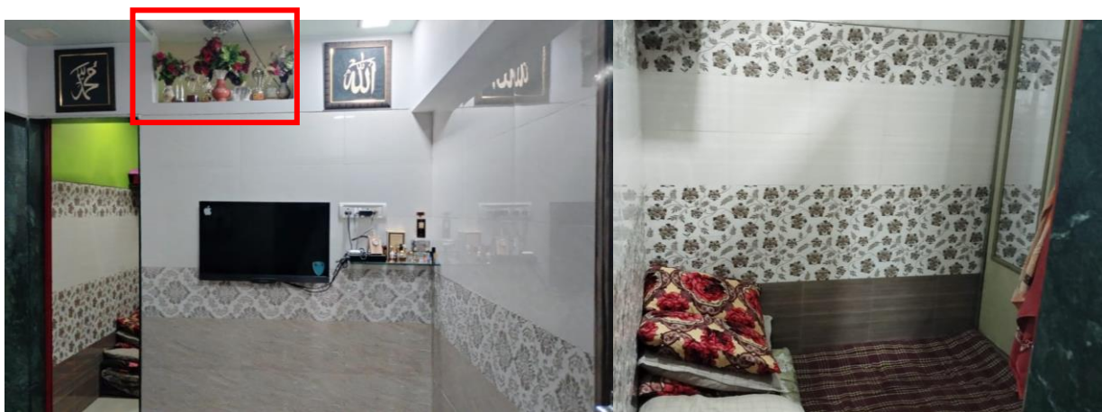
Figure 21: Wall separating bedroom & hall; Source: Research Assistant (RA)
