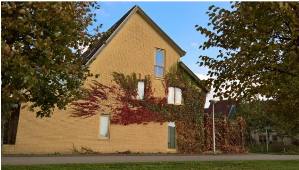
Figure 32 Green walls covering some buildings act as insulation.
