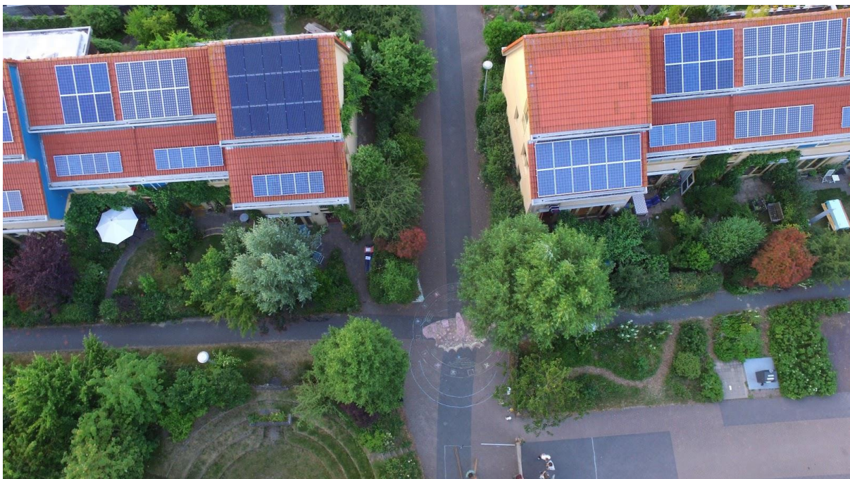
Figure 33 Aerial view of De Kersentuin showing solar panels on the roof.
