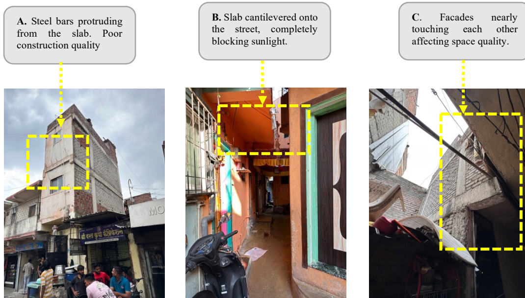
Image 18: Construction quality of incremental additions in Netaji Nagar. Source: Author (2023)
