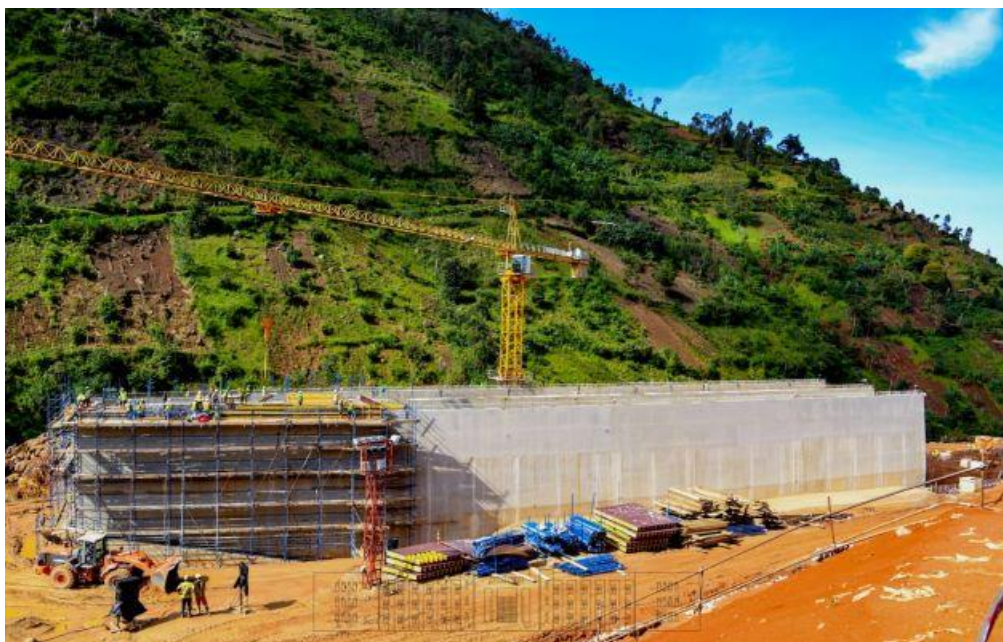
Figure 2: Jiji-Mulembwe Hydroelectric Power Site During Construction of the Dam
