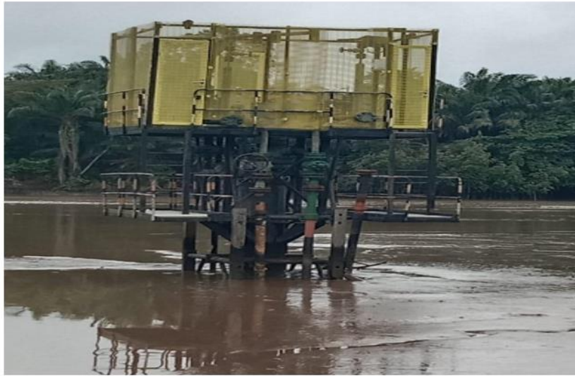
Figure. 4.2: Oil exploration facility on a polluted water body (creek) in Ugborodo community Source: Author
