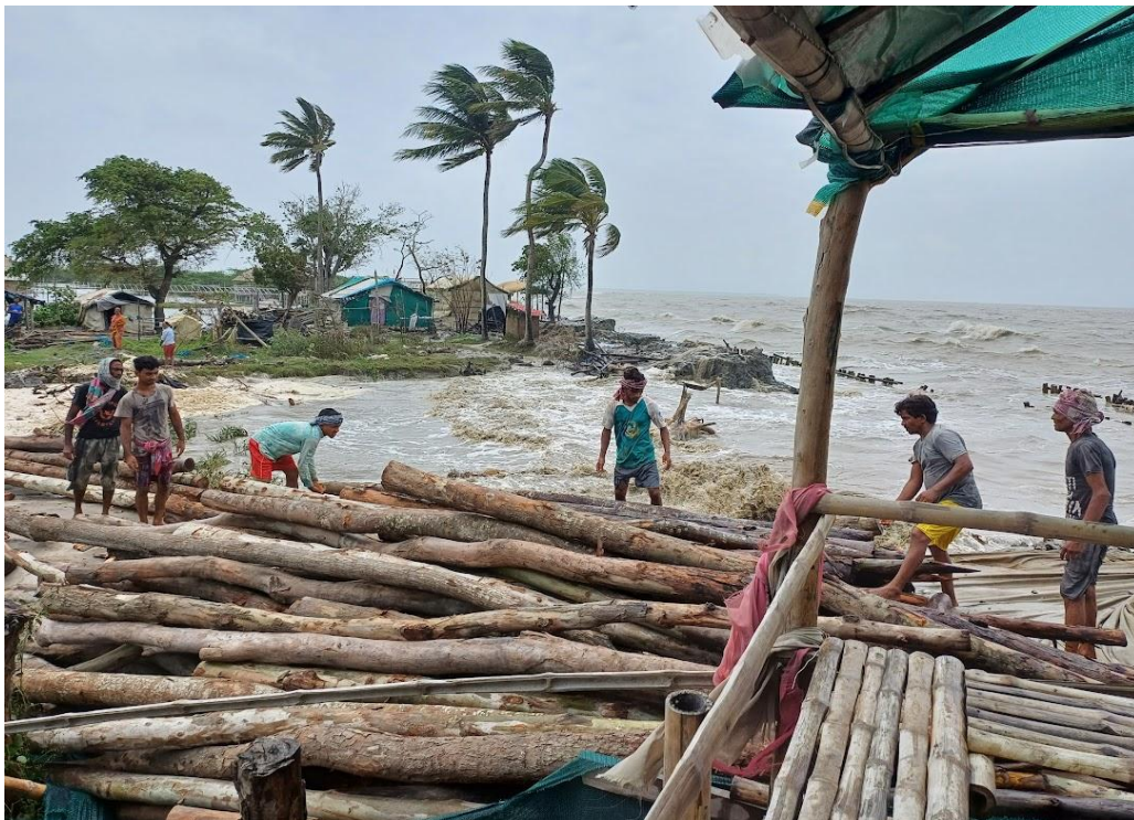
Figure 2. Islanders of Mousini trying to rebuild the embankment that keeps the gushing water at bay Source: Photo taken during fieldwork (5 July, 2023)
