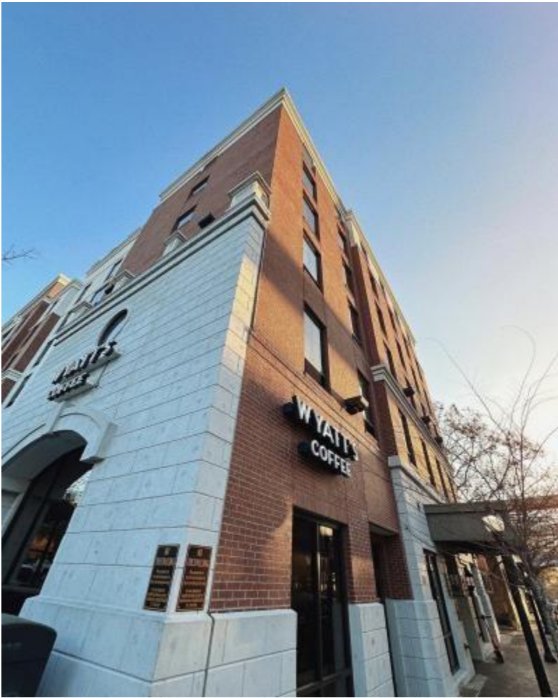
Control Condition Image
