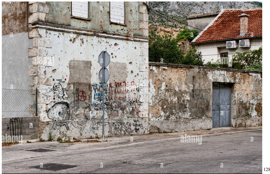
Figure 3. Damaged buildings from the Bosnian War in Mostar, 2011.
