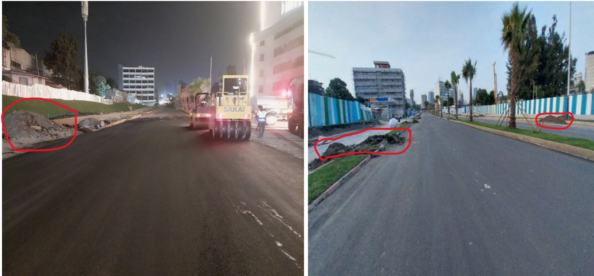
Photograph 4 Field view of the Mexico Roundabout to Sarbet project site
