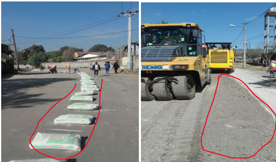
Photograph 3 Field view of the Kagnew Roundabout to Egypt Embassy project site
