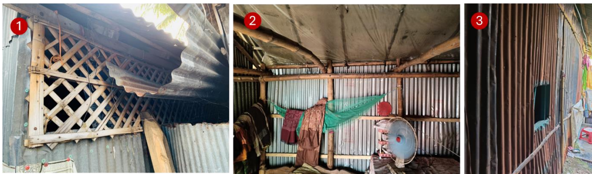
Figure 14: Facade modification for ventilation (Source: survey, 2024).
