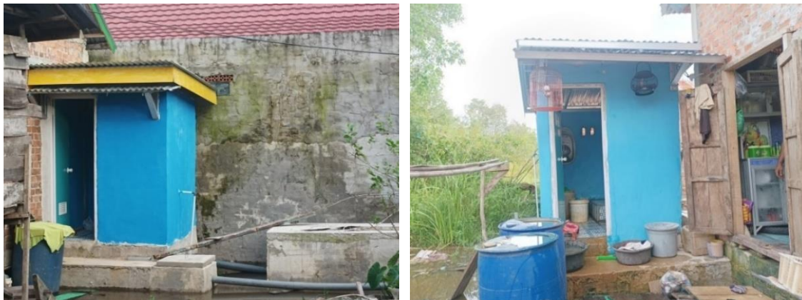
Photograph 12: New individual toilet installation
