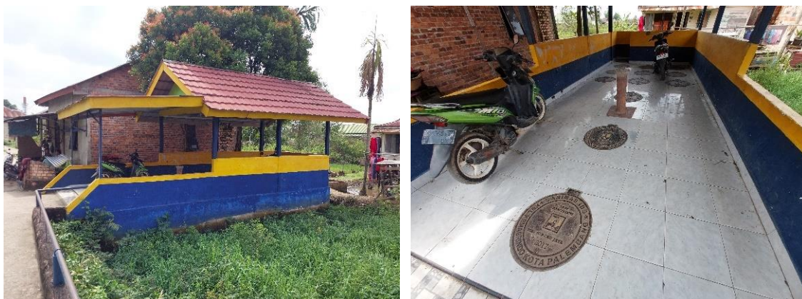
Photograph 13: Communal wastewater treatment plant
