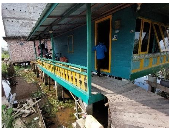
Housing structure upgrades from wooden to a concrete pile, they kept the stilt house typology.
