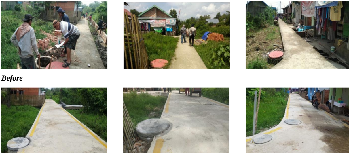
Photograph 2: Sanitation facilities upgrades
