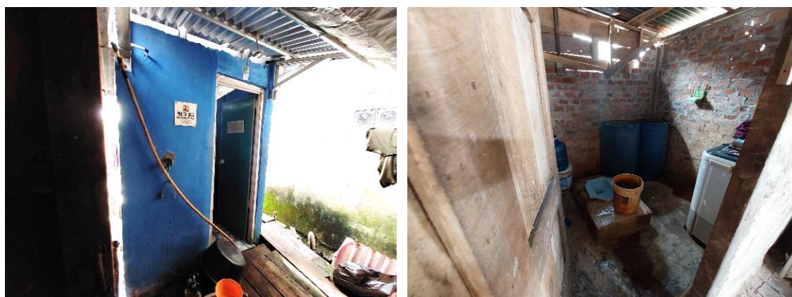
Photograph 11: Existing individual toilet improvement
