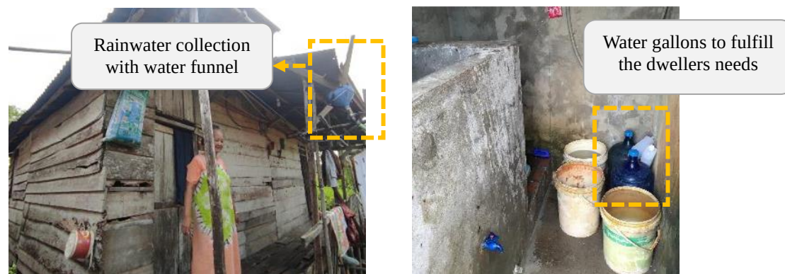
Photograph 1: Example of water collection before upgrades
