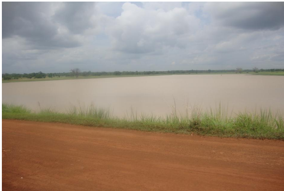
Figure 2.1 The Karni Dam
