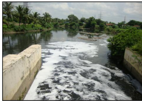
Figure 1.3: Drainage water coming to EKW
