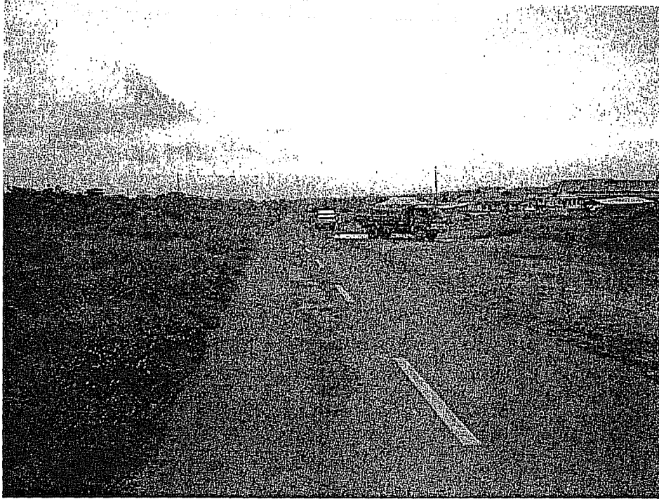
Figure 9 Main road project in Saumlaki town
